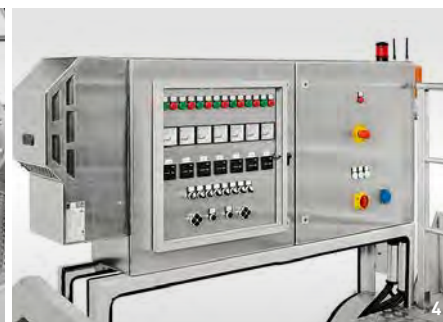
4 Thanks to an integrated cooling unit, the cabinet is designed even for the warmest ambient temperatures. In an emergency, the ground sludge remover can also be controlled directly via the explosion-proof switch unit.
